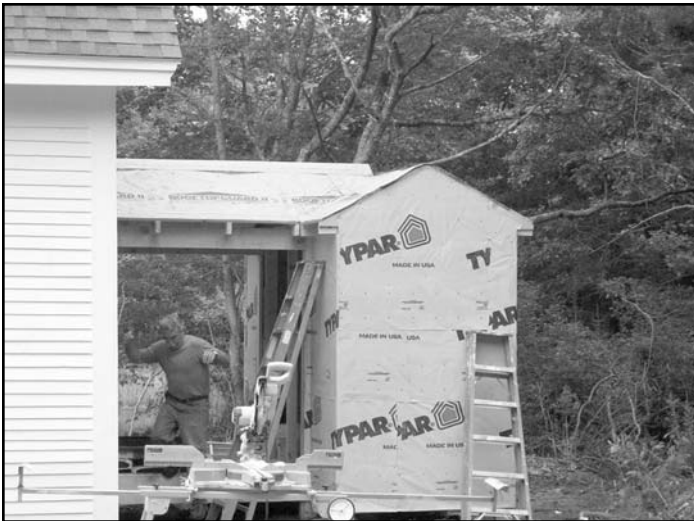
Privy rebuild gets started...
