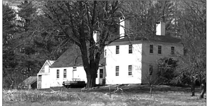
The colonial Cape structure (left-side) of Sproul Homestead was likely built in the mid-18th century when the 100-acre property was first deeded to Robert Sproul.
