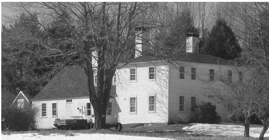
The Sproul Homestead on Rte. 129: two-story Federal main house (1815) attached in 1833 to center chimney Cape (1749) at the rear.
